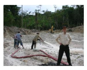
Figure 9- The laborers are spraying water to the alluvial sand
